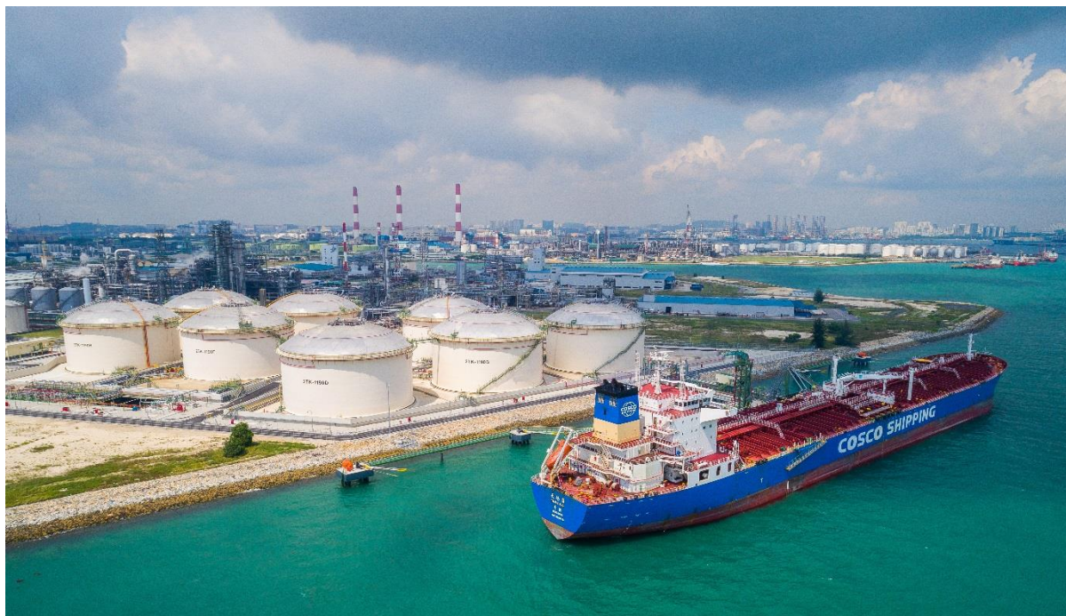
PCS Naphtha Import Facilities successfully commissioned on 11 November 2017. Berthing/unloading of its 1 st vessel "Tian E Zuo".
